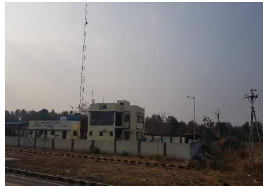
Toll Building at Km.382+920
