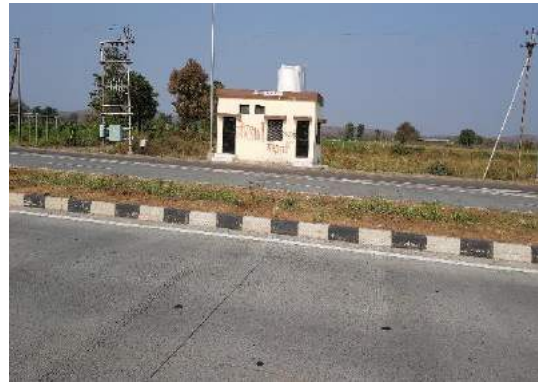
Truck Lay bye at Km.384+300
