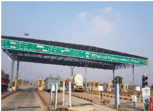
Toll Plaza at Km.382+920
