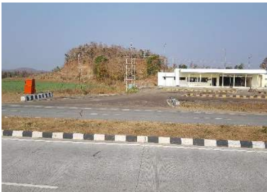
Rest area at Km.385+300
